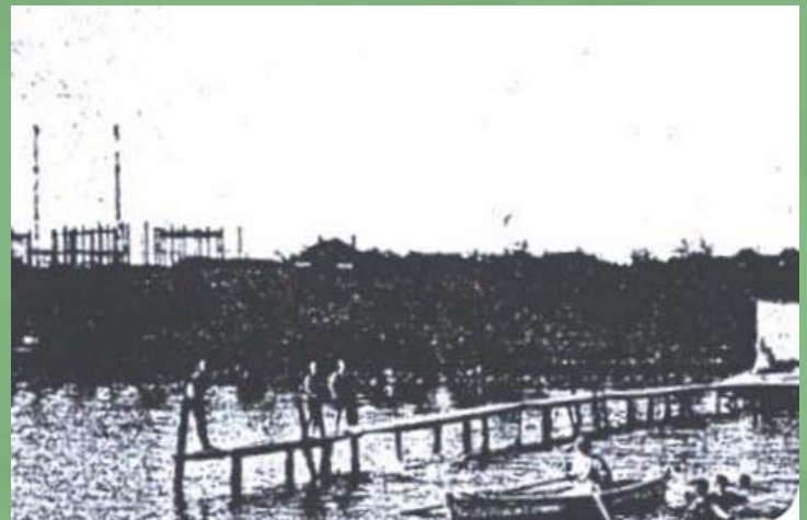
Figure 2 The steel structure of the original building can be seen in the left corner of this old picture.
